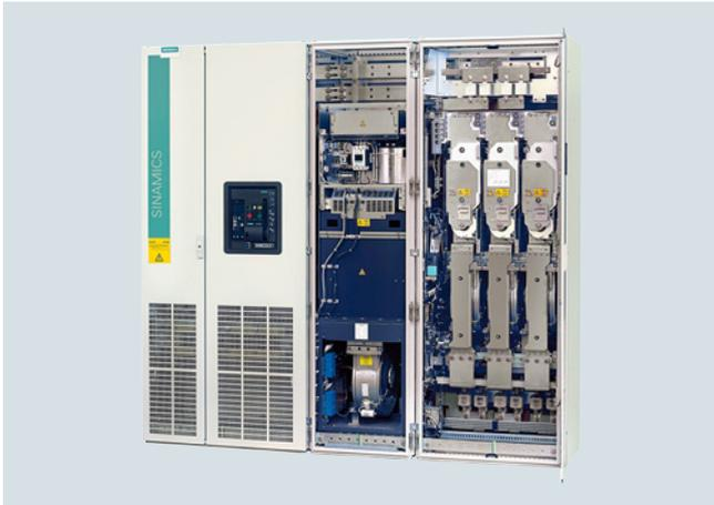
Active Line Modules are regulated infeed/regenerative units. They can supply energy to the DC link and return regenerative energy to the supply system.
